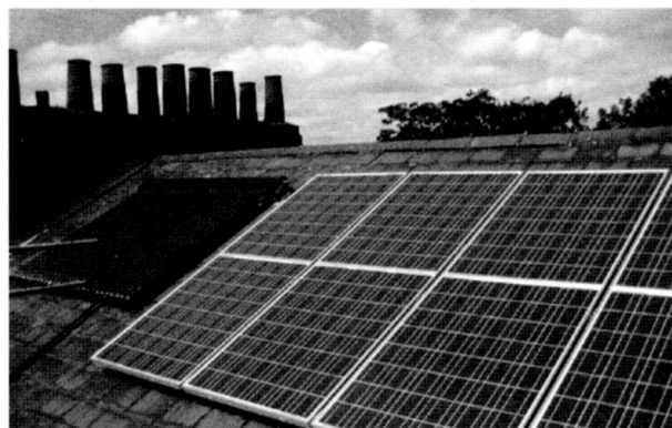
Photovoltaic and solar thermal panels at the back (east facing) of a Highbury Place house.
